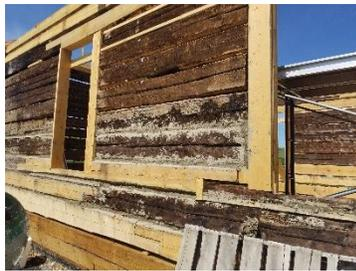
working steadily throughout the summer. The early stages of the project saw the timbers salvaged from the fire put into place and then the clay chinking pressed into place to create a seal. The roof and walls were next, and we were finally able to see the building in place on the horizon. In early August work began on the bell tower and the
